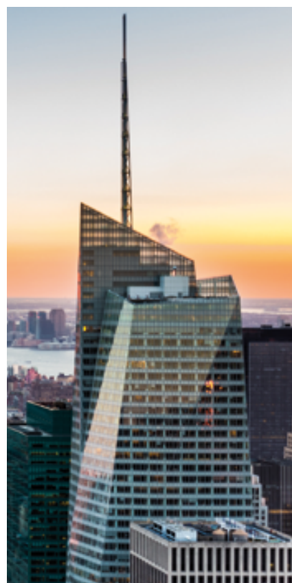
Fot. 3. Bank of America Tower w Nowym Jorku, USA (fot. © mandritoiu – stock.adobe.com)
