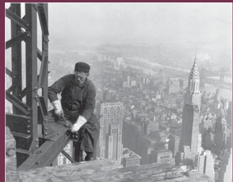
Budowa Empire State Building (fot. Wikipedia)
